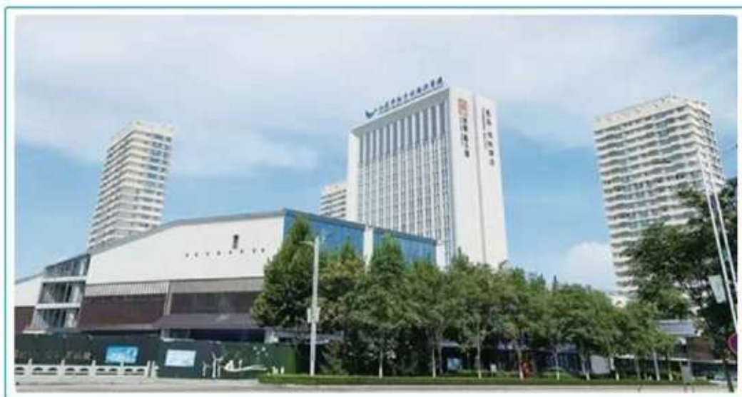
Ningyang Lvjing Xintiandi Residential Power Distribution Construction Project
