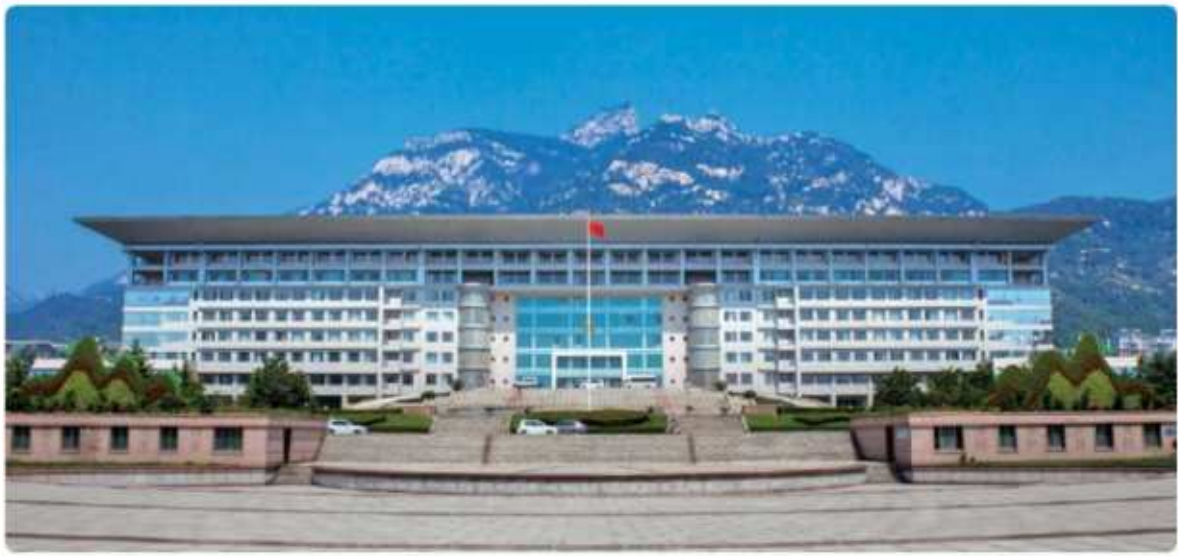
Tai'an Housing and Urban Rural Development Bureau Leigushi Street Middle Section Renovation Project (Fuqian Street 10KV Distribution Room Power Relocation Project)
