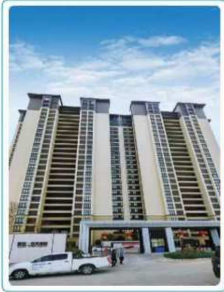
Jimei Jiayueju Power Distribution Construction Project in Tai'an City
