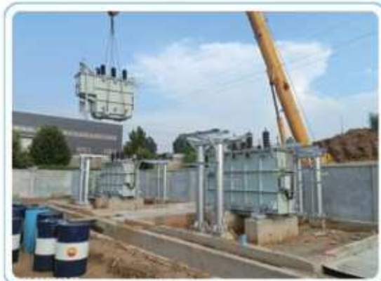
Jinan Yingcheng Intelligent Manufacturing Industrial Park Power Transmission and Transformation Project SZ20-12500KVA/35kV Transformer Procurement
