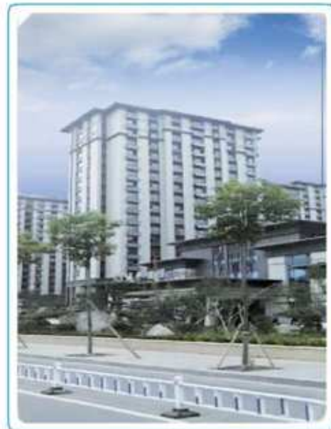
Xintai City Kaiyuyuan Residential Power Distribution Construction Project
