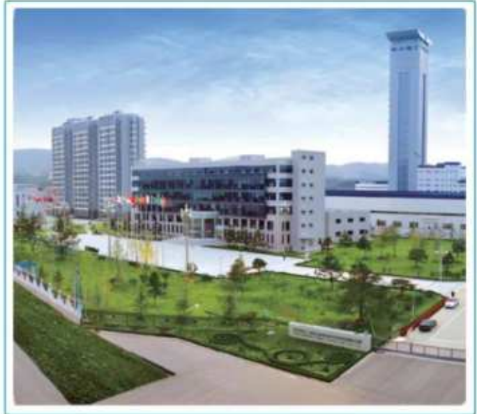
Xintai Tebian Electrician Lu Cable Company's 14th Five Year Plan for Power Distribution Civil engineering and electrical installation
