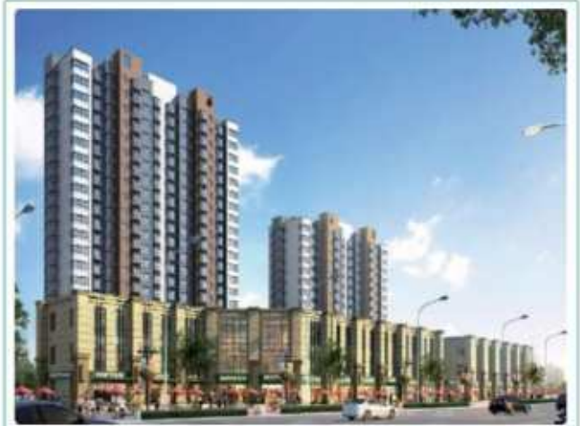
Power Construction Project of Wuzhongbei Commercial Residential and Financial Building in Qingyun County
